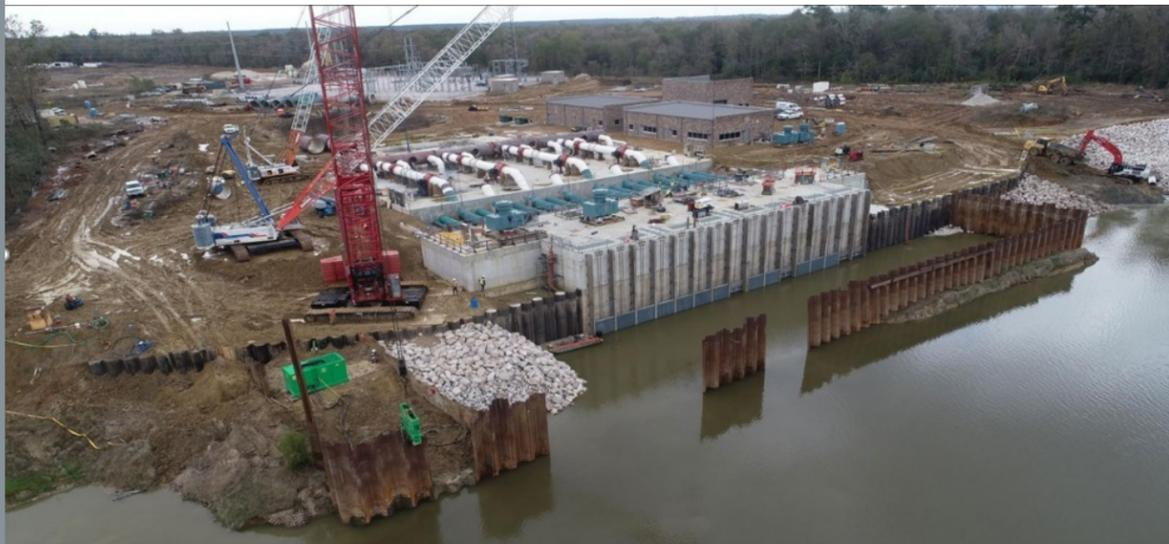
Pictured above: The dam that held back the Trinity River for over two years is being removed, revealing the pump intake station.
