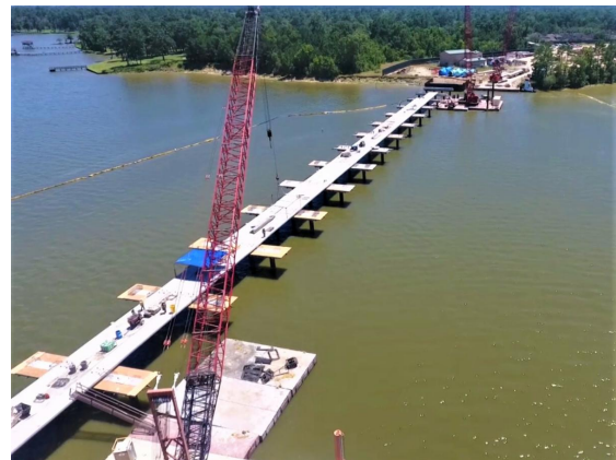
NEWPP Influent Pump Station Bridge
